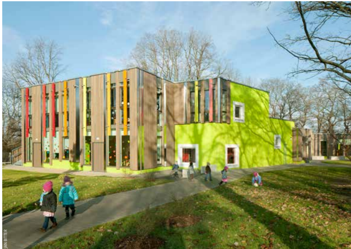
↑ KINDERGARTEN LICHTENBERGWEG, LEIPZIG Susanne Hofmann Architects developed a new child-care centre through an intense participatory planning process, which has provided differentiated indoor and outdoor spatial experiences and learning environments since 2012.
