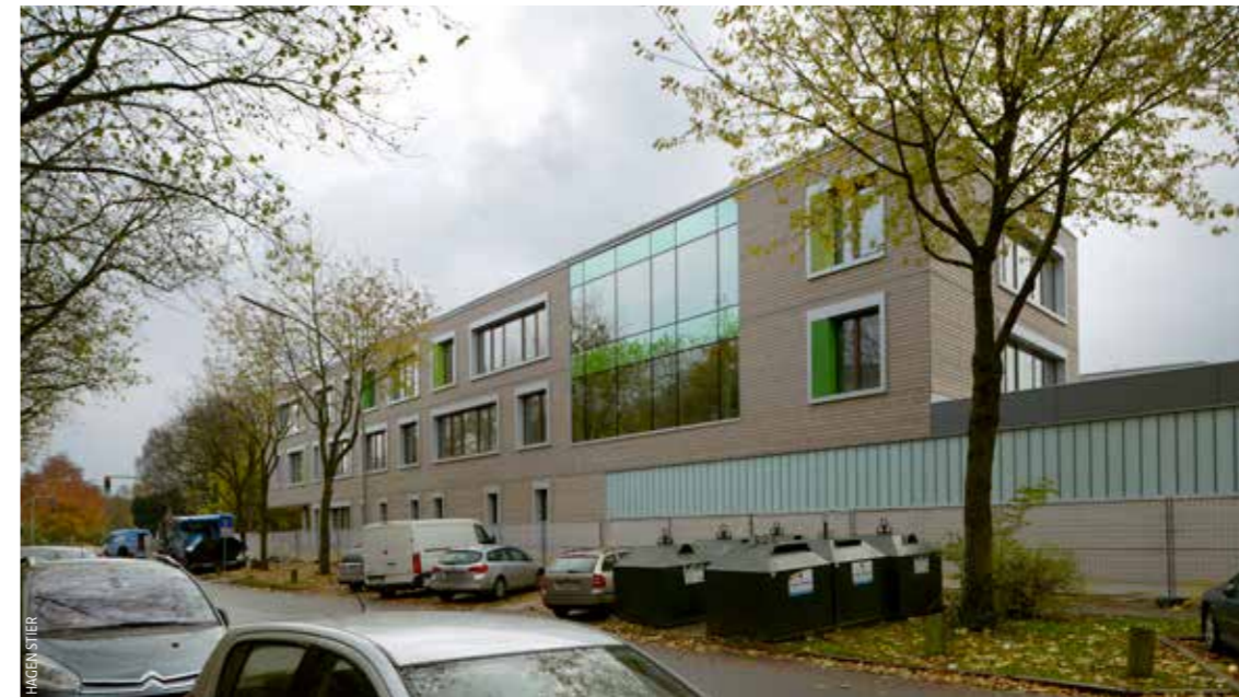
↑ TOR-ZUR-WELT EDUCATIONAL CENTRE, HAMBURG Within the context of the Hamburg International Building Exhibition 2013, bof architects won a competition with a project that transformed a collection of multi-generational educational institutes into a coherent educational landscape. They used wood as the main facade material, which is untypical for site and function, and created unique classrooms by playfully applying polygonal forms to the facade and interiors.
